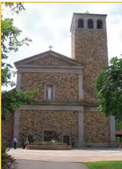
Main entrance of the Shrine Church.
